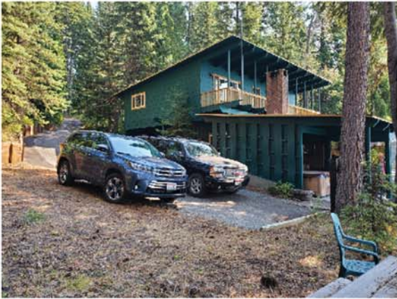
EXISTING HOME: WEST FACADE
