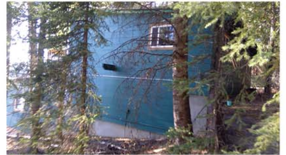
EXISTING HOME: EAST FACADE
