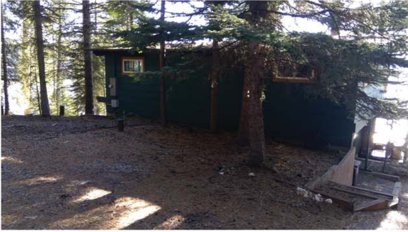
EXISTING HOME: NORTH FACADE
